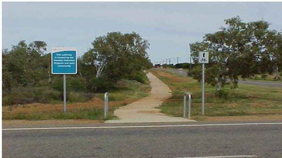
Figure 2 - Boor Street, Carnarvon
